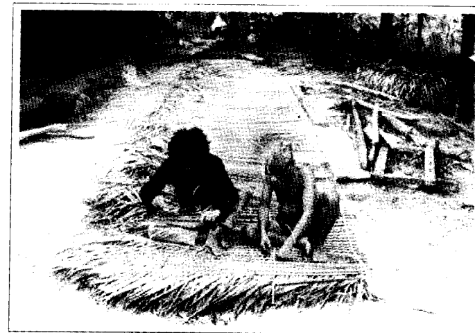
Making rattan wattle for house-roof
