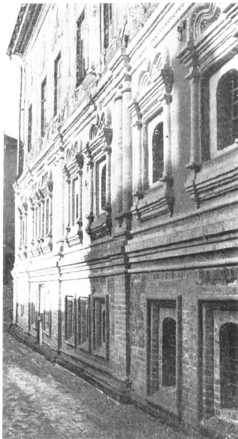
42. Palace of the Boyar Troyekurov. End of the 17th century
