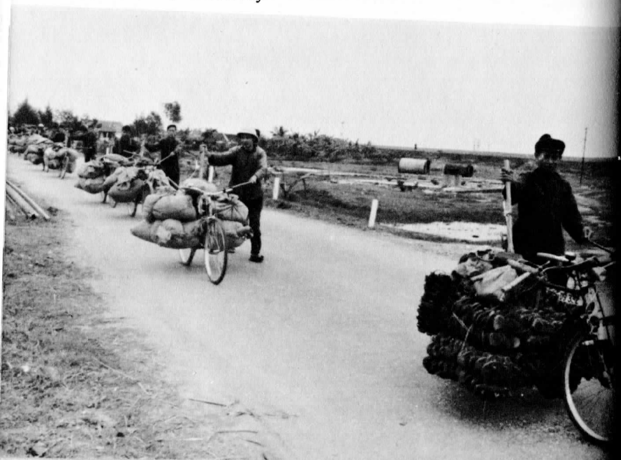
12 Bicycles, reinforced with bamboo tubing, could carry up to half a ton of supplies twenty miles a day
