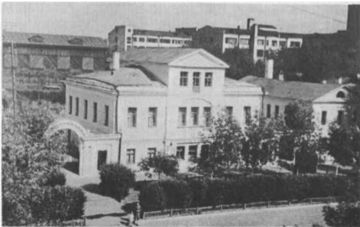
Yekaterinburg: building which housed the clandestine Party school (1905); now the Sverdlov museum
