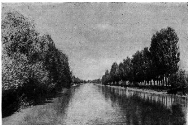
A section of the Stalin Great Ferghana Canal in the Central Asian Republic of Uzbekistan
