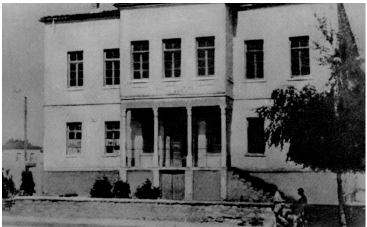
The Korça National Lyceum's dormitory building.
