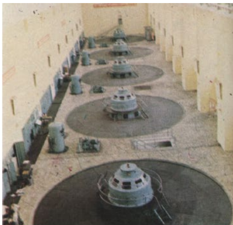
View of the dam under construction at the «Enver Hoxha» hydro-power station at Koman, which will be the most powerful of Albania
