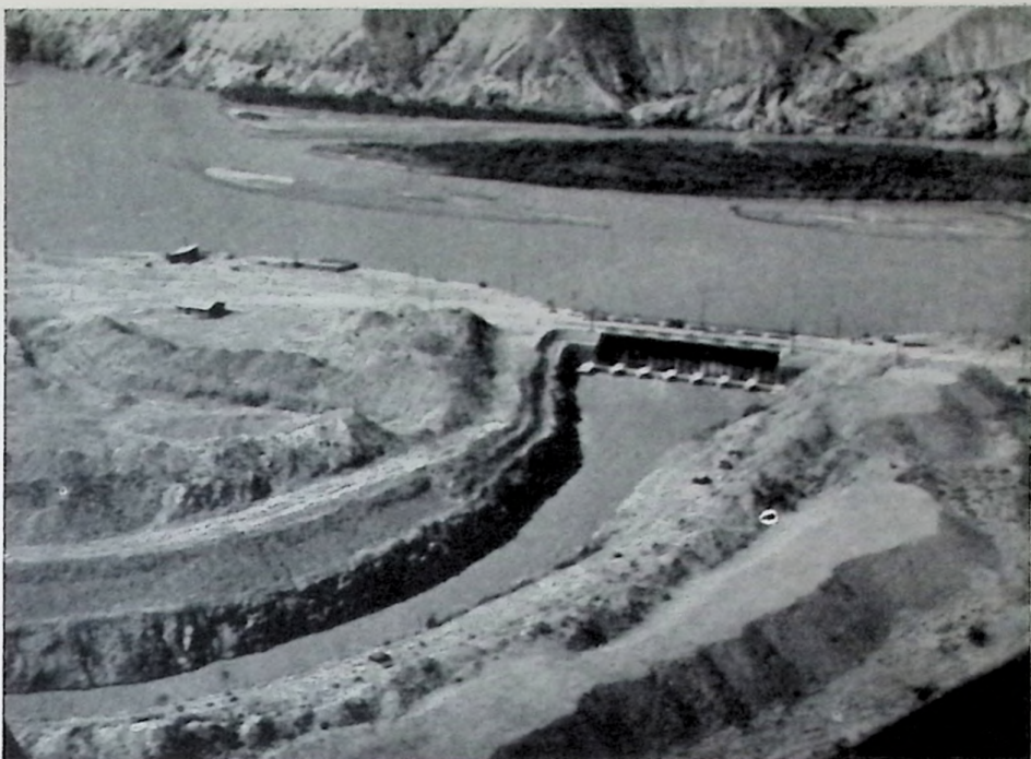
IRRIGATION—Aerial view of the Vakhsh dam and of a canal leading from it. Irrigation projects constructed in Soviet times increased the Republic's agriculture sixfold.
