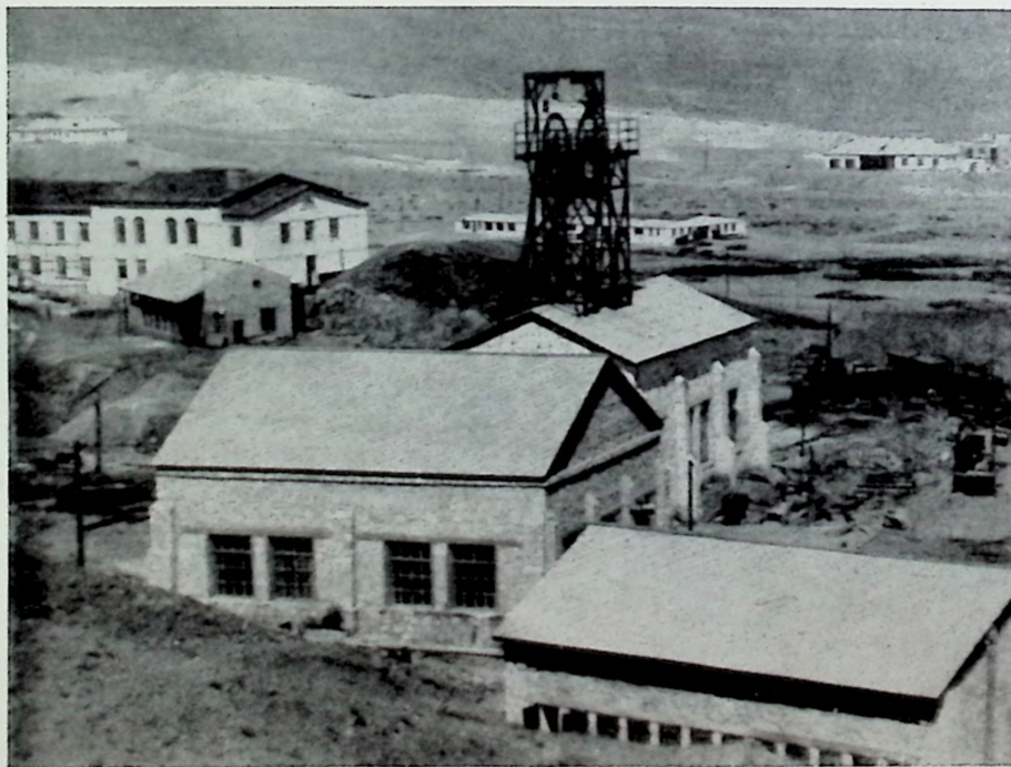
COAL INDUSTRY—Buildings of the coal fields in the Isfarlinsky district of the Tajik Soviet Socialist Republic.
