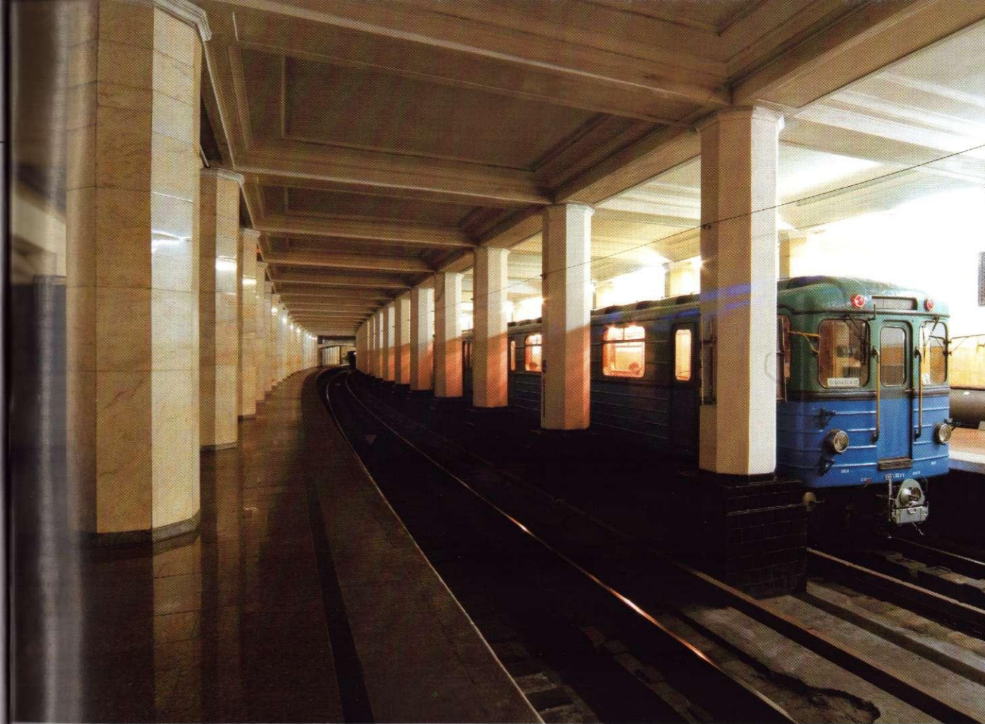
Alexandrovsky Sad. The only underground station in Moscow with side platforms.
