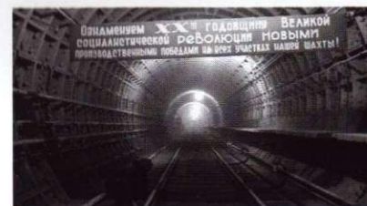
At the building of the second phase of the metro
