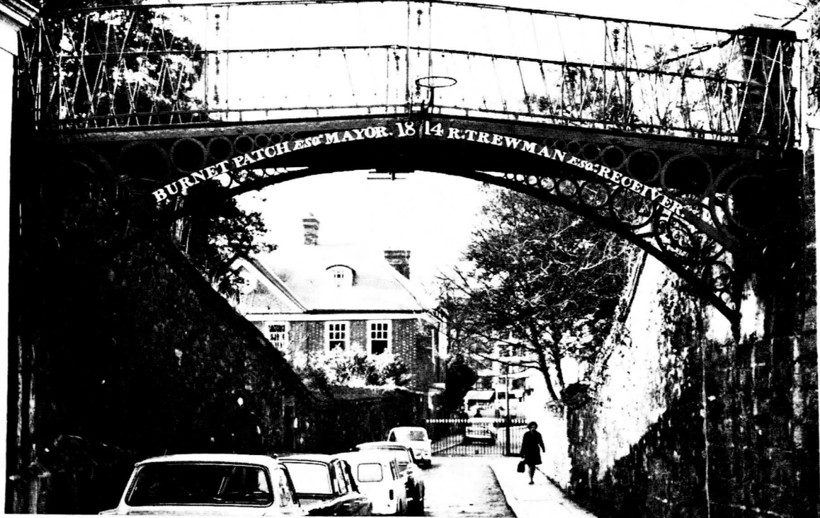
14 Iron Footbridge, The Close, Exeter
