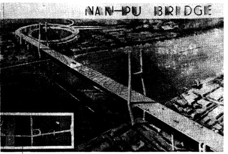
A mock-up of the Nanpu Bridge across the Huangpu River. The bridge, now under construction, will be a six-lane, 8,346-metre span under which 40,000-ton ships will be able to pass when it is finished. It will play an important role in the development of Pudong.
