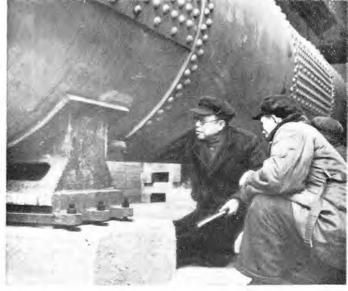
Technicians making a final check on the vat for processing rot-resistant railway sleepers in the first lumber mill to be built with such equipment in China. The mill, in Hanyang, will shortly start production
