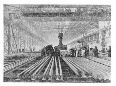
The new heavy rolling mill produces its first batch of heavy steel rails
