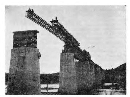
Work proceeding on the recently restored railway bridge over the Yongjin River on the Sinmak-Kaesong section. Korean and Chinese railwaymen are working side by side rehabilitating lines, bridges, stations and trains in North Korea
