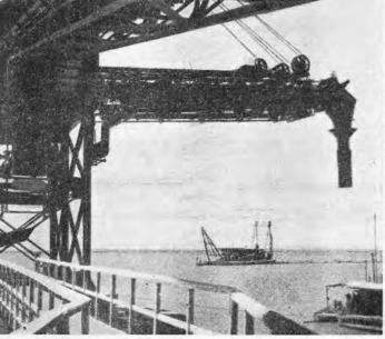
The new port of Hsinkang near Tientsin is one of the world's largest sheltered ports and will be the main ocean gateway to North China. Our picture shows a mechanical coal transporter for fuelling ships in the port
