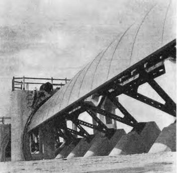
This 1,054 metres long movable dam at Taipingkou with 54 sluice gates controls the flow of water into the Yangtse flood detention basin—it is the biggest dam in China
