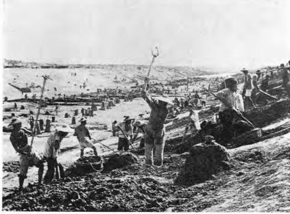
Peasant builders are removing 25,000,000 cubic metres of earth from the bed of the Sui River, part of the vast Huai River control project to protect one-seventh of China's arable land from flood
