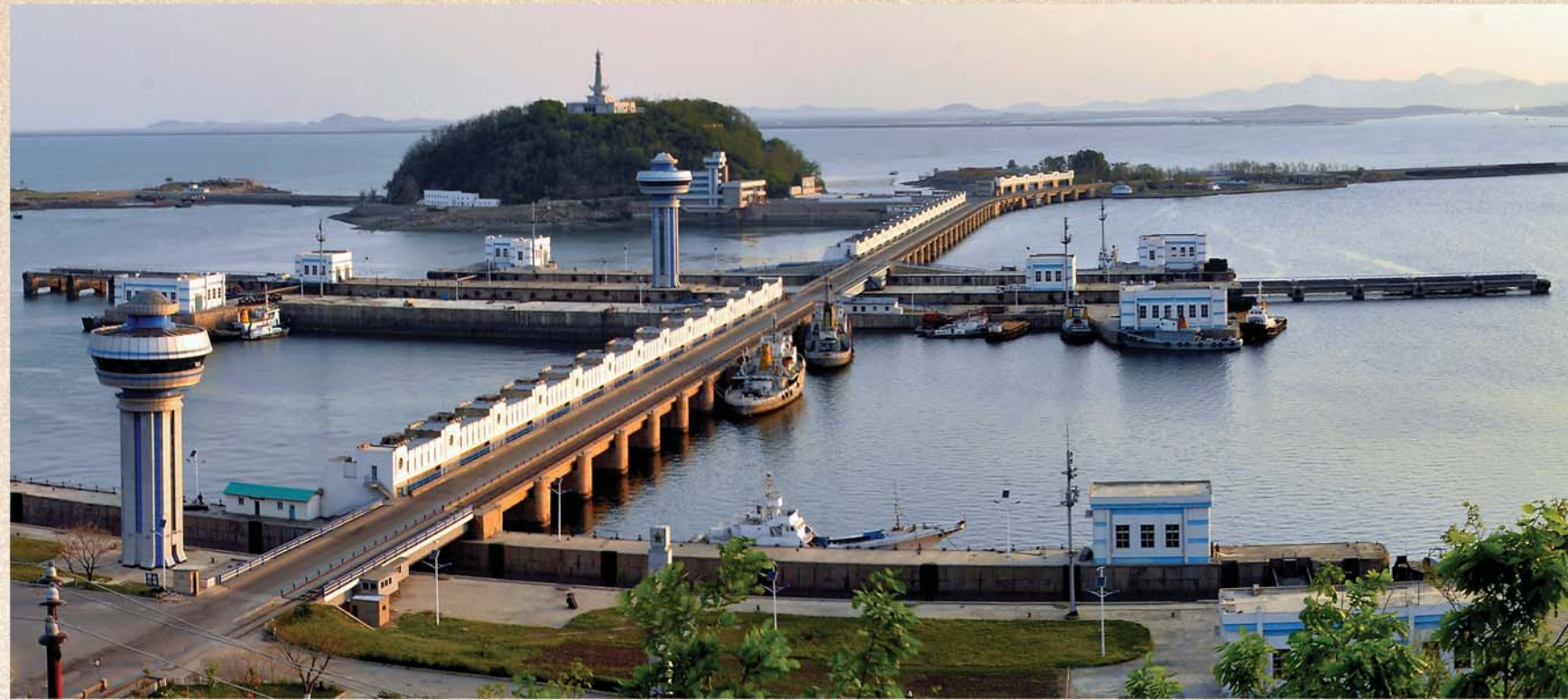
The 8km-long West Sea Barrage was built in five years.
