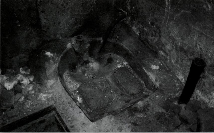
Some of the bunkers were fitted with rudimentary sanitary facilities for the crew. This example has two marks for the soldier to place his feet. The hatch to the side would have been covered. (Author's photograph)
