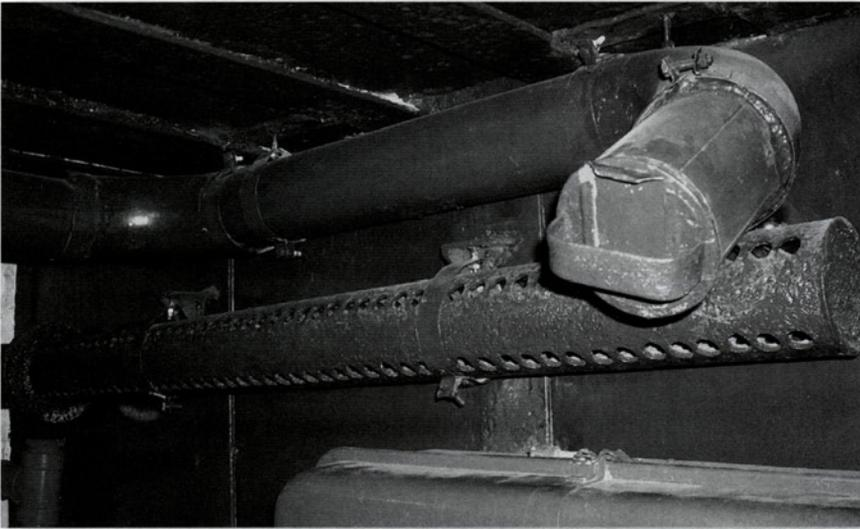
Fumes from the generator room were extracted through a pierced pipe and vented outside the shelter. However, the system was not found to be particularly effective and was later changed. (Author's photograph)
