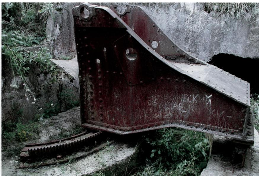
This position near Tarasovka in the Kiev Fortified Region originally mounted a 76.2mm M1900 gun (now removed) on a Durlbacher caponier mount. This was an open position also known as a TAUT position. (A. Kainaryan)
