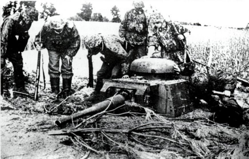
An emplaced T18 tank with 45mm gun is inspected by SS troops in the distinctive splinter pattern fatigues. Camouflage that would have disguised the position lies strewn around. This turret was installed in the Stalin Line and was captured in the summer of 1941. (J. Magnuski courtesy of S. Zaloga)
