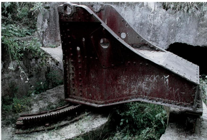
This position near Tarasovka in the Kiev Fortified Region originally mounted a 76.2mm M1900 gun (now removed) on a Durlacher caponier mount. This was an open position also known as a TAUT position. (A. Kainaryan)
