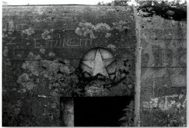
The entranceway to a bunker in the Polotsk Fortified Region. These were constructed in 1930 when there was less pressure to complete the work and unusually the builders have taken the time to include a Soviet star above the door. Also just visible are the impressions from the shuttering boards and the internal loophole. (Author's photograph)
