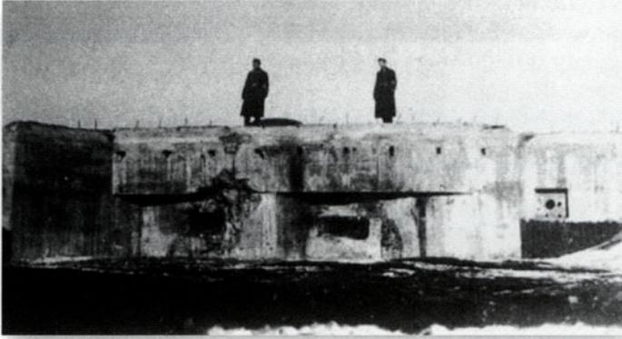
Two German soldiers stand atop a captured bunker of the Molotov Line. The embrasures were damaged in the fighting to break through the Przemysl Fortified Region. Just visible between the two soldiers is the top of the armoured cupola. (T. Idzikowski)
