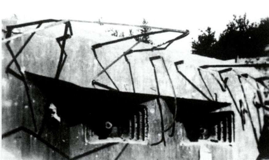
A bunker of the Molotov Line armed with two 76.2mm guns. Clearly visible are the armoured housings, which were stepped to reduce the damage from ricochets. The iron framework protruding from the top of the bunker would have been used to secure camouflage. (T. Idzikowski)
