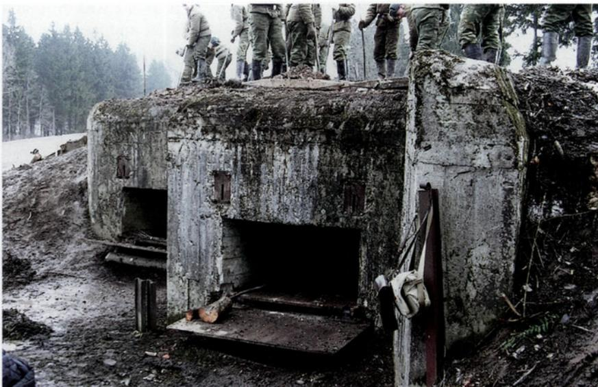
Soldiers help to clear artillery bunker No. 134. This was later fully restored and now forms part of the Stalin Line Museum at Zaslavl near Minsk. Even at this early stage of restoration it is possible to see the armoured shield and opening for the winch cable. (E. Hitriak and I. Volkov)
