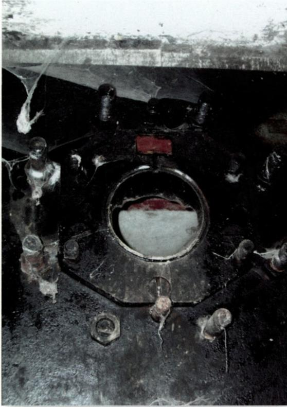
To provide close-in fire support small openings were let into the side of the bunker. These were fitted with armoured plates that could accommodate the 7.62mm Degtyareva light machine gun. This example was in a bunker in the Przemysl Fortified Region of the Molotov Line. (Author's photograph)
