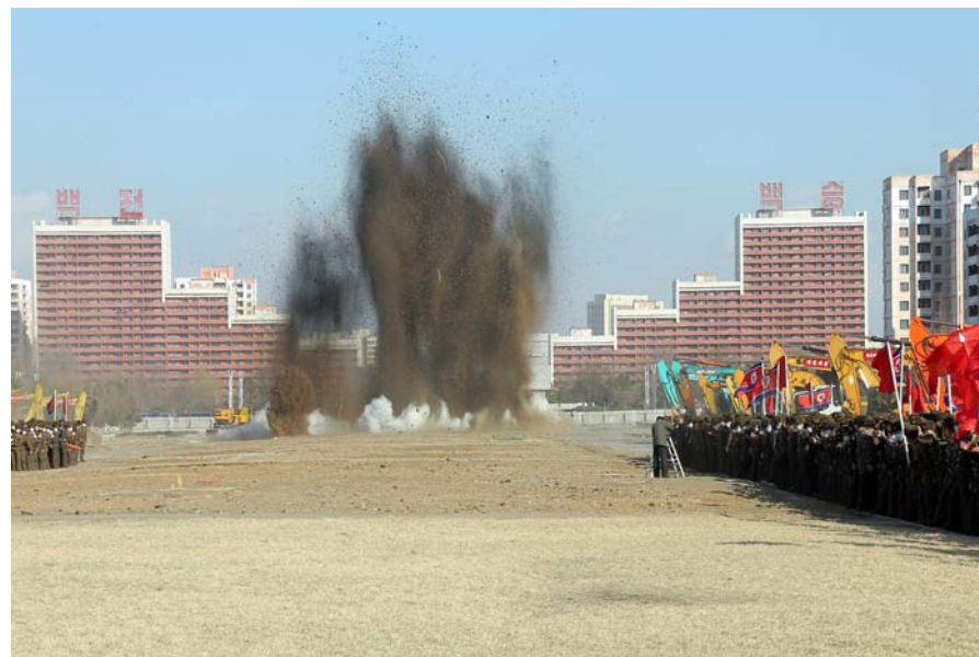
Ground-breaking ceremony of the Pyongyang General Hospital
