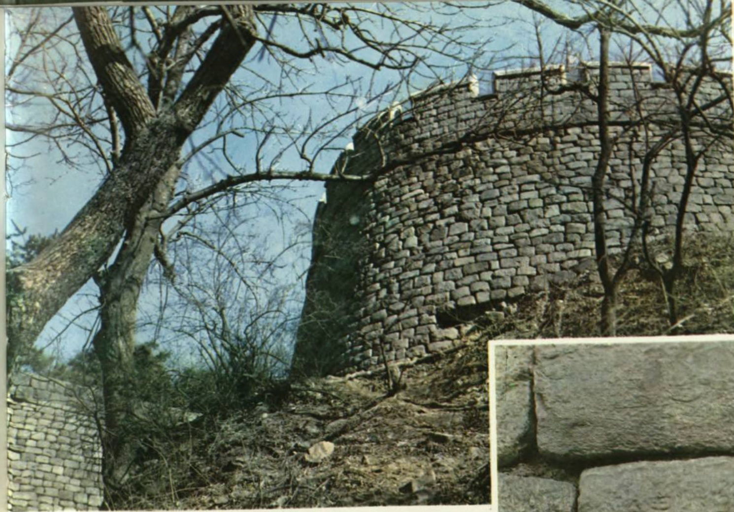
The outer wall of the Chilsong-mun Gate
