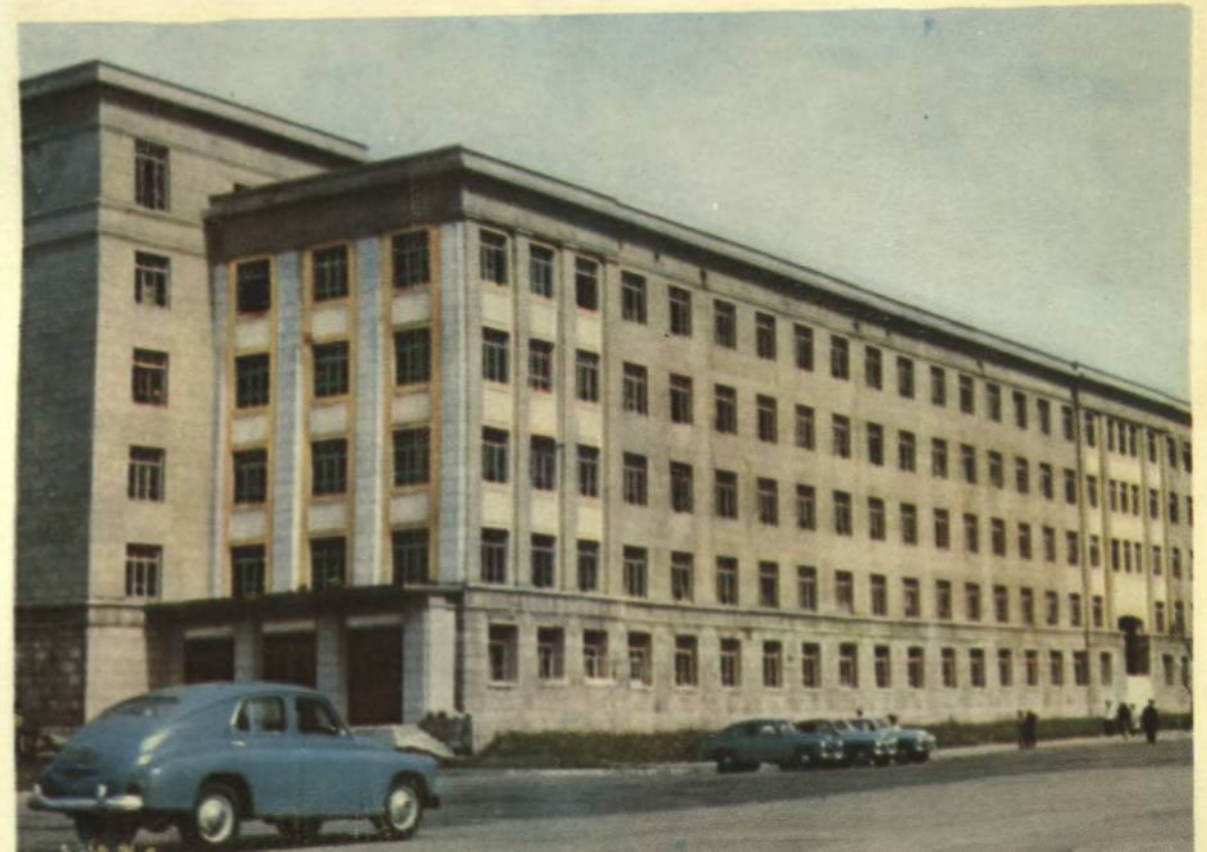
Newly erected Government Building No. 3
