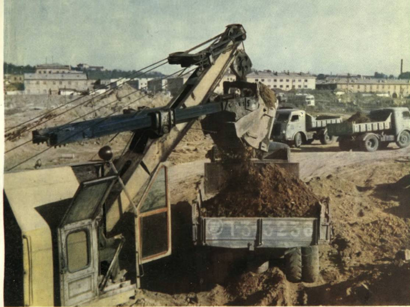
River-dyke project at Kamhyun-dong
