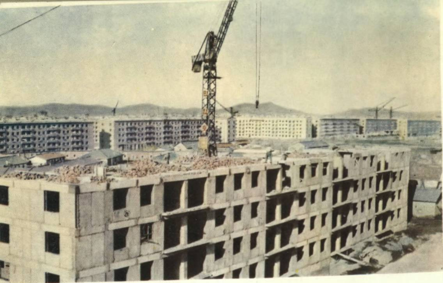
A construction site in the Botong Plain
