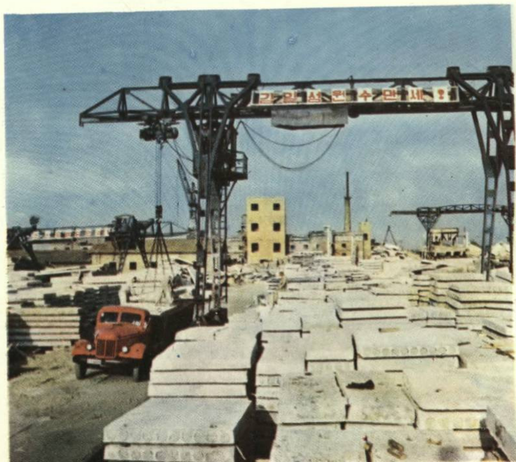
The Pyongyang Concrete Block Factory. The factory turns out blocks in large quantities to step up the construction of the city
