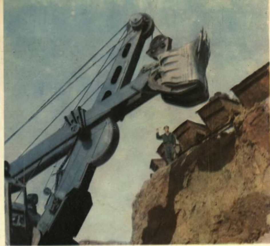
Excavating clay at the Daisung Brick Yard
