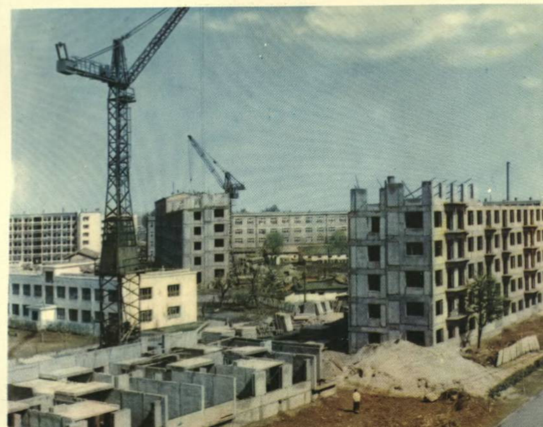
New apartment buildings under construction in East Pyongyang
