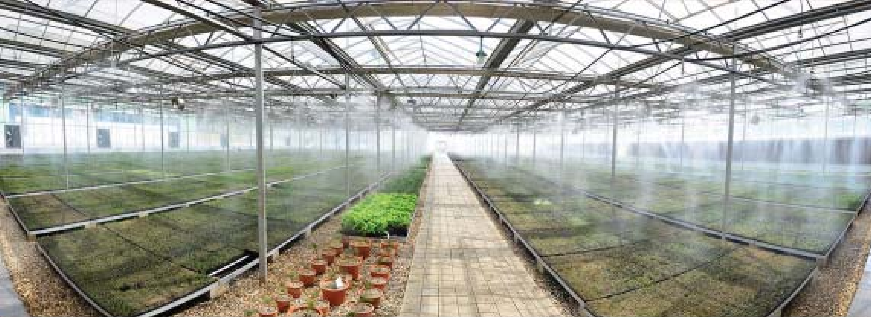
An efficient integrated control system has been established to provide the most suitable conditions for the cultivation of saplings including temperature, humidity, sunlight, content of carbon dioxide, ventilation, irrigation and application of nutritive solution
