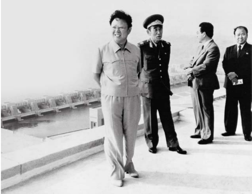
Kim Jong Il inspecting the West Sea Barrage (June 23, 1986)
