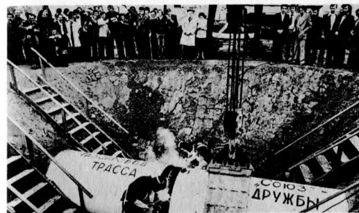
Welding the final joint of the international gas pipeline at the Soviet-Czechoslovak frontier.
