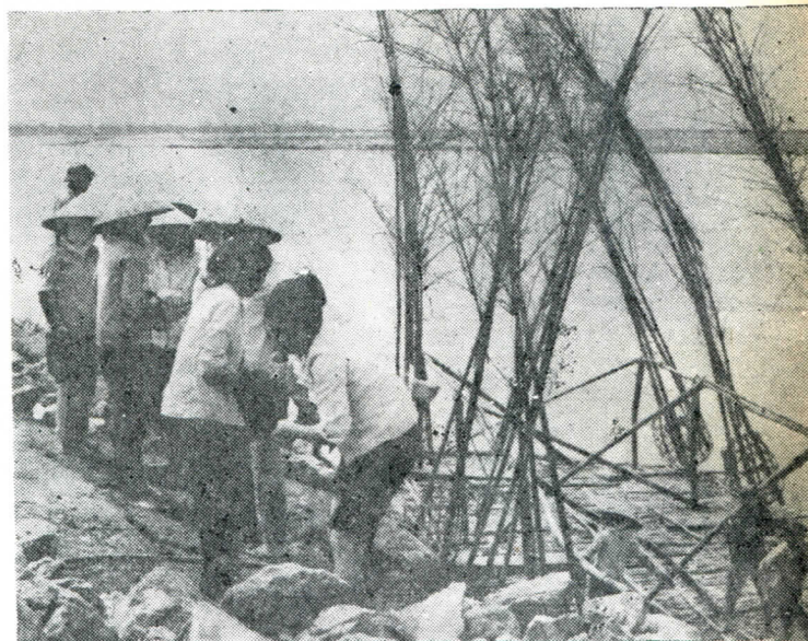
Building a culvert to stop sea-water in Phu My (Tien Giang province).
