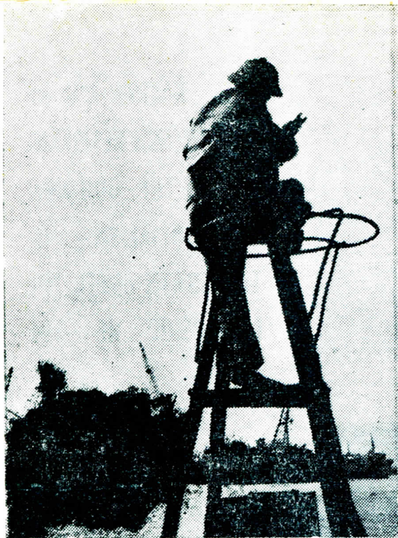
Insulating electricity in Haiphong port
