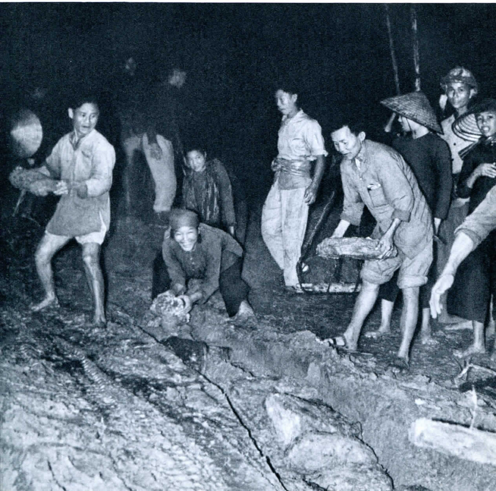
Roads damaged by enemy bombing are repaired at night to ensure smooth passage of supplies
