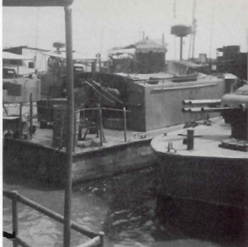
This ASPB has had the original single machine gun mount replaced by a twin mount. Note how the guns can receive ammunition from both sides. Unfortunately while the twin .50 caliber machinegun mount gave the Vietnamese a tremendous amount of firepower its range often led to civilian casualties outside the immediate battle area which did little to endear the Vietnamese Navy to local inhabitants. (Mesko)
