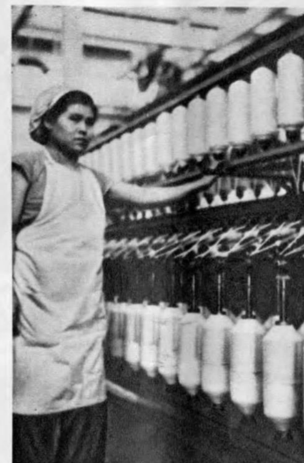
COARSE SPINNING —the rovings are set on an intermediate frame and spun into coarse yarn
