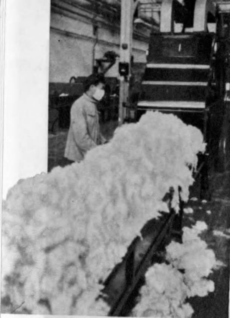
SCUTCHING —raw cotton is fed into the scutcher, to be cleaned of all broken seeds, grit, and other impurities
