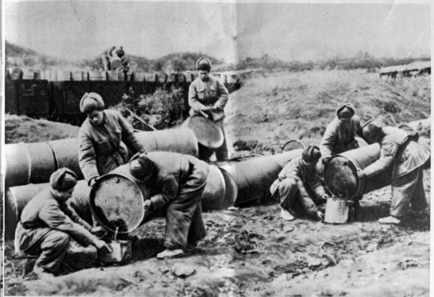
Even the empty oil drums from the front are drained before being returned to the rear. The oil is filtered and stored for use
