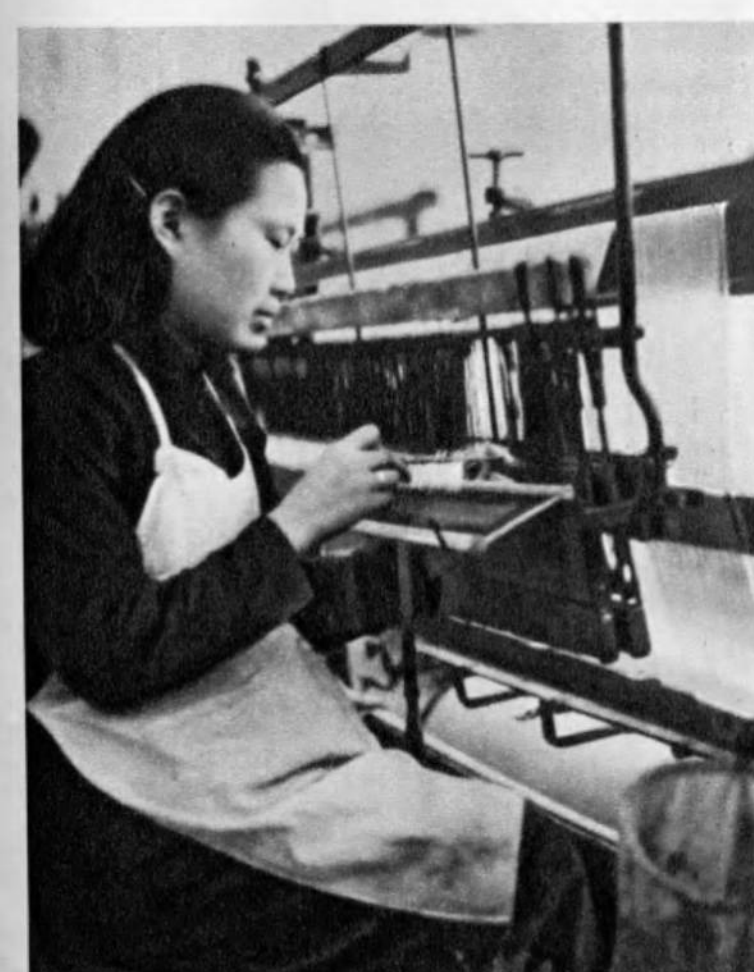
HEDDLING —the warp threads are guided through the heddle eyes to the lathe of the loom
