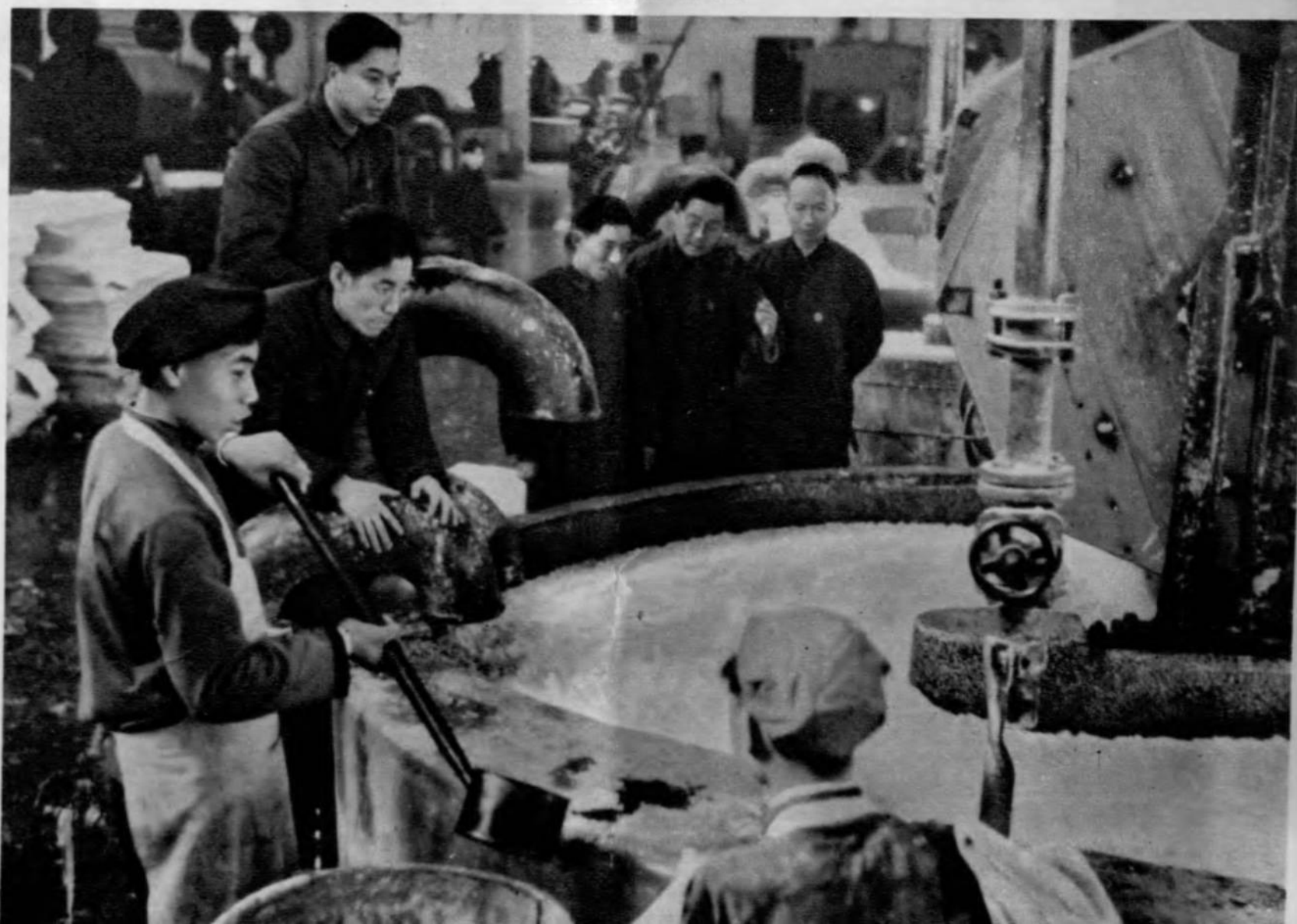
Engineer Liu Hsien-tseng, chief-engineer Chiang Feng-shu and technician Li Yen-fen of the Tientsin Paper Mill, who overcame the problem of shortage of timber pulp by evolving a method of pulping grass
