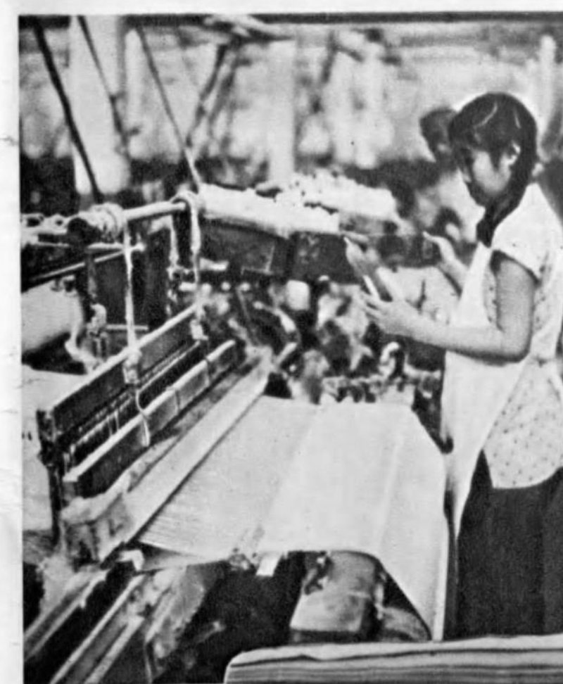
WEAVING —a reed separates the warp threads and beats up the weft threads, weaving the yarn into cloth
