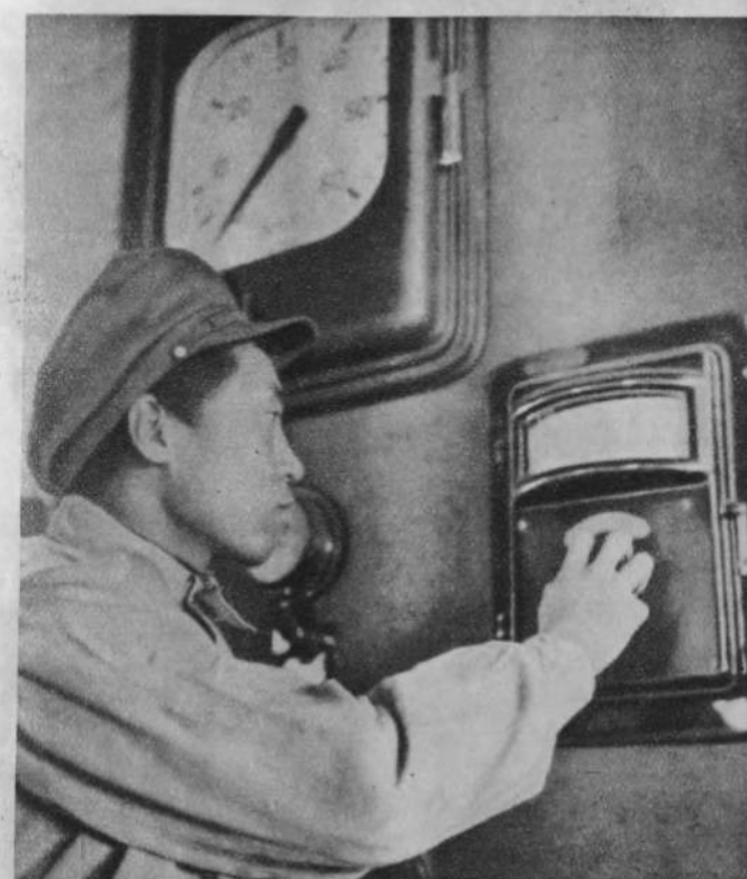
A careful check is kept on the temperature of the generator
