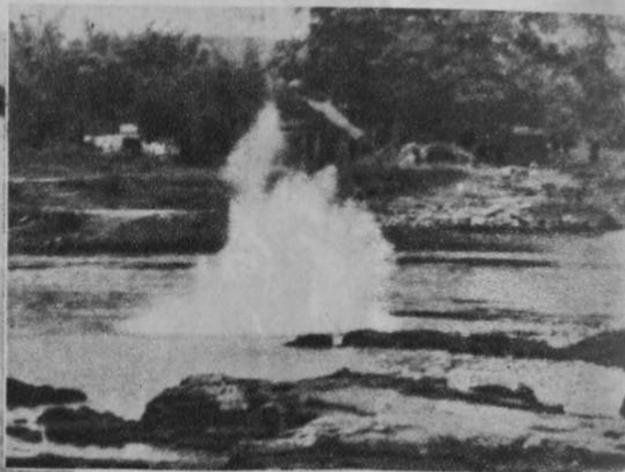
Dangerous reefs in the Pearl River estuary, which have been the cause of many shipwrecks in the past, are now being demolished by the Pearl River Water Conservancy Administration.
