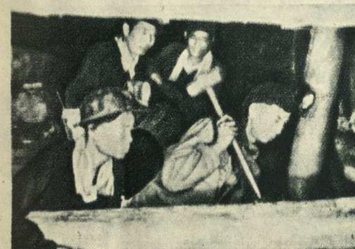
The use of pneumatic drills in coal-mining must be closely co-ordinated with the work of propping, shovelling and transport.
