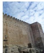
The openings along the sides of the Wall are the putlog holes which are marks from the scaffolding used for its construction.
